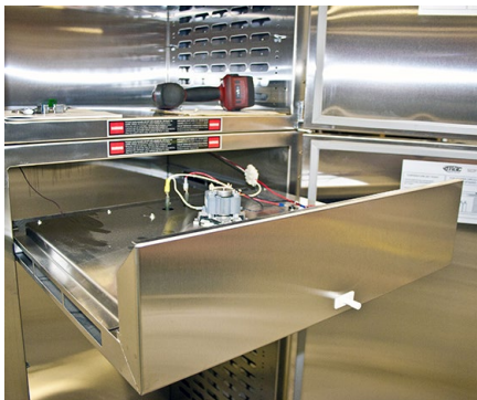
Fig. 3: Lower Drawer Assembly - Dual Cabinet
